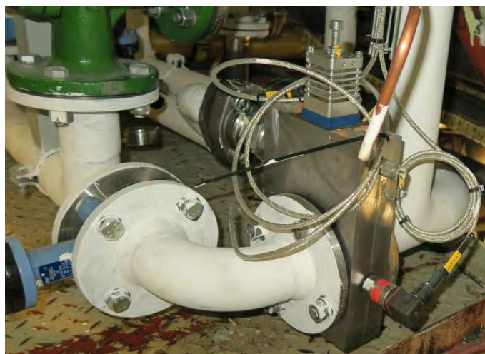
Picture 14: Fuel pressure sensor at booster pump
